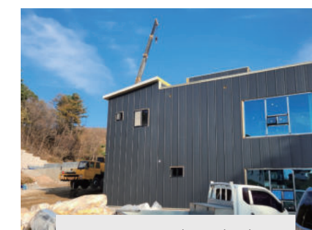
tennis court Electrical and communication construction photos
