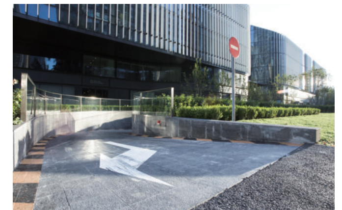
Underground parking lot entrance/exit
